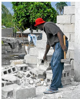
Worker removes debris from the Clinic's second floor collapse.
