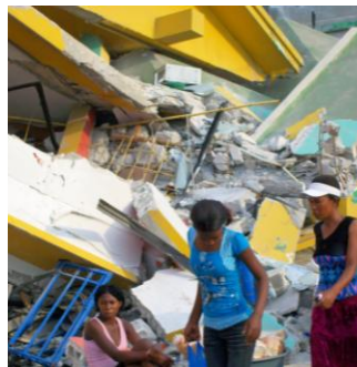
Signs of the earthquake are everywhere.
